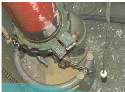
Building site pumps
